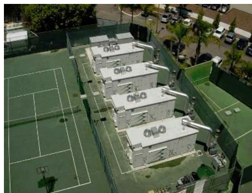
Figure 2: Sheraton San Diego's clean and quiet fuel cells are located next to the hotel's tennis courts
