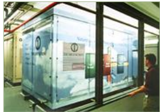
First National Bank of Omaha's fuel cells provide high quality, reliable power to their data processing facility
