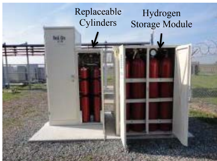
Figure 4. Example ReliOn fuel cell system with replaceable cylinders and an HSM [11]
