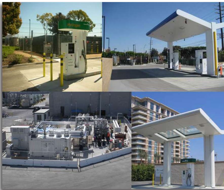
Air Products' Various Filling Stations and ADG Facility (Bottom Left)
