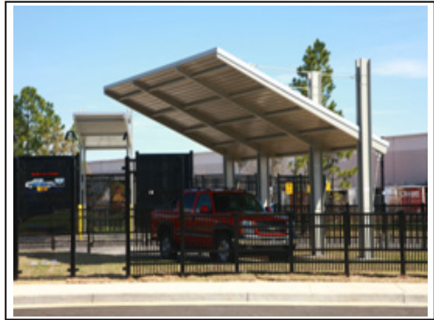
Figure 17: Sage Mill refueling station, SC
