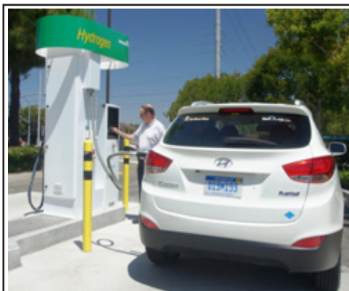
Figure 16: A customer fills up on hydrogen derived from renewable biogas at the Orange County Sanitation District, Fountain Valley, CA. The hydrogen is dispensed from the Energy Park built by Air Products.
