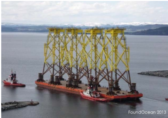
Fig. 2.5.7 – Traditional vertical transport of RWE jackets.
