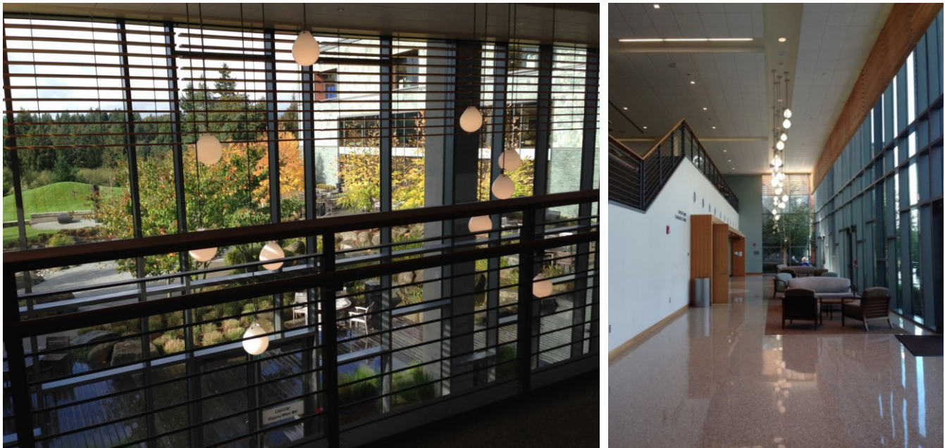
Figure 1. Pendant globe luminaires are lamped with vertically-oriented Lunera ® Helen lamps. The diffuse, even light is a characteristic of both the vertical lamp and the luminaire itself. Photo credit: PNNL.
