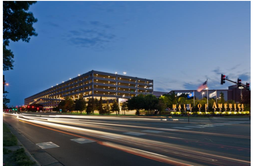
Mall of America Parking Garage New lighting: 0.076 W/sf Saving: 7 million kWh annually
