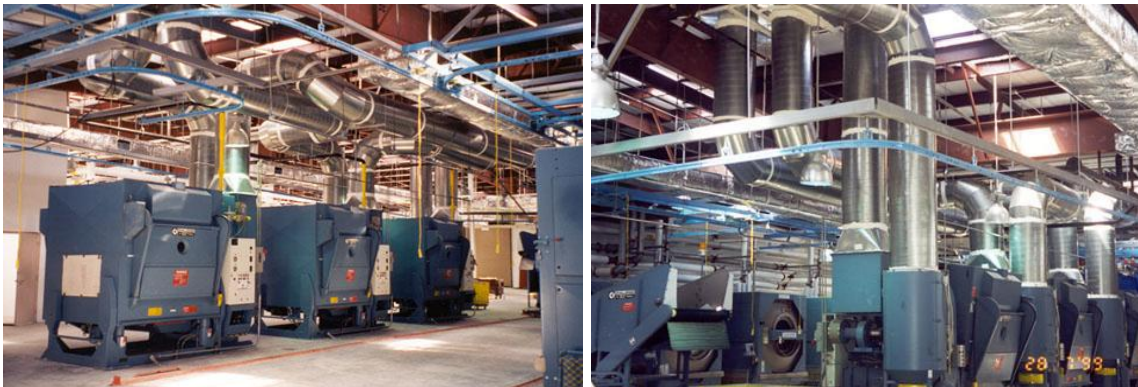
Figure 8-4: Off- Premise Laundry Facility Featuring The Largest-Capacity Washing And Drying Equipment
