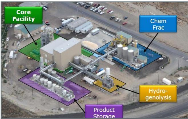
ZeaChem, Inc., has successfully constructed and operated a 10 ton/day integrated biorefinery in Boardman, Oregon, with assistance from a \$31.25 million
