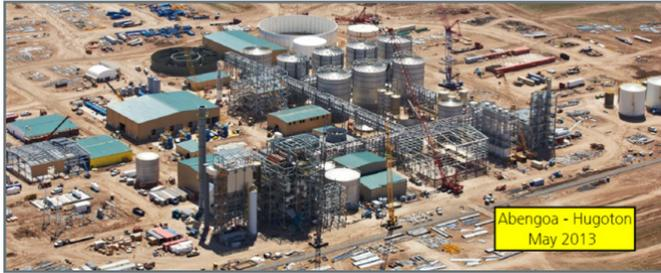
Abengoa Bioenergy Biomass of Kansas, LLC, is in the process of designing and constructing a biorefinery facility to produce cellulosic ethanol in Hugoton, Kansas. The process utilizes an enzymatic hydrolysis process to produce ethanol, process steam, and all electrical power required to operate the facility via an integrated biorefinery and cogeneration system. Initial feedstocks that will be used are corn stover and wheat straw, with other
