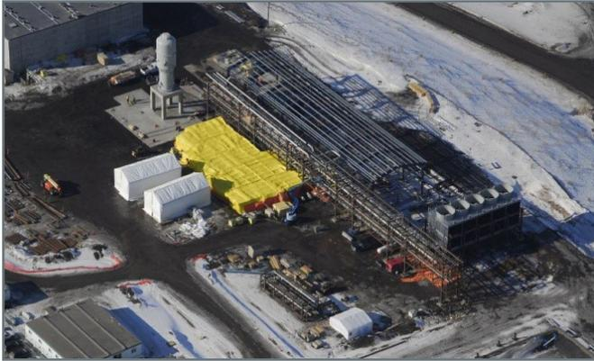
Enerkem will build and operate an MSW-to-biofuels plant in Pontotoc, Mississippi, that will convert 100,000 dry tons of sorted MSW and other locally sourced residual woody biomass into 10 million gallons of RFS2-compliant cellulosic ethanol annually. The project will produce a renewable fuel from a non-food, sustainable source (MSW) that will reduce dependence on foreign oil, increase the life of existing landfills, and lower
