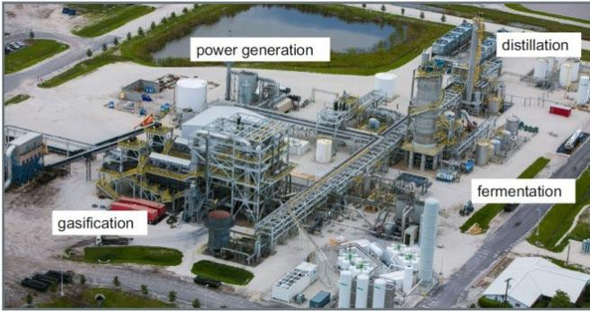
INP BioEnergy has completed construction and commissioning and is now starting operations of the first commercial-scale facility employing the INEOS Bio bioenergy process technology on a site in Indian River County Florida (known as the Indian River BioEnergy Center). The facility will produce eight million gallons per year (mgpy) of cellulosic ethanol and 6 megawatts (gross) of electricity at full rates. The project is demon-
