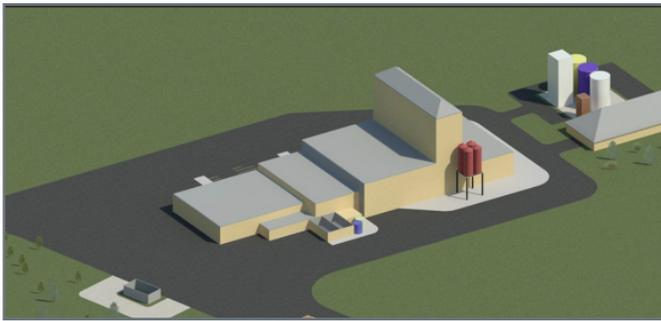
Proposed Plasma Gasification Waste-to-Energy Demonstration-Scale project. 180–200 tons/day of biomass waste resources (municipal solid waste). This project will output clean, renewable energy in the form of synthetic gas, steam, biofuel or electricity, and vitrified non-leaching solid by-products. The project is located near an energy host in International Falls, Koochiching
