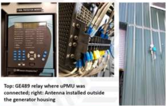
microPMU Installation at Eyak substation – Main Town feeder
