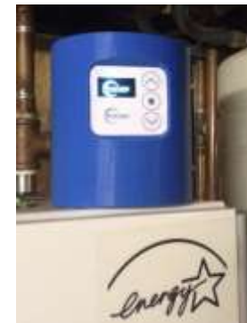
Packetized Energy's connected thermostat for water heaters
