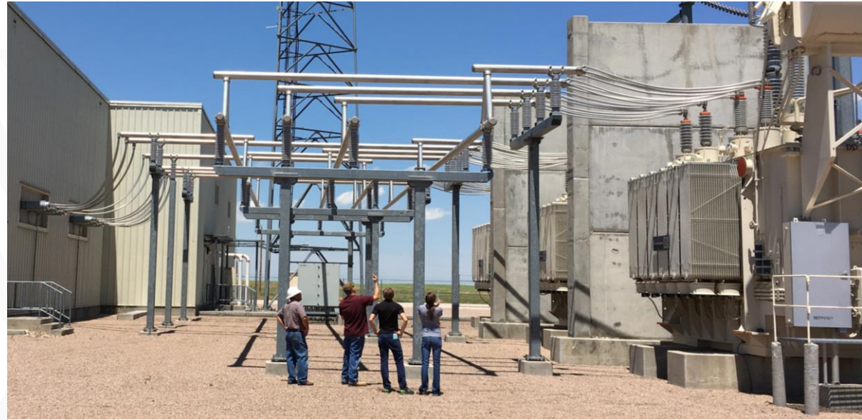
NREL and SPP tour WAPA's Virginia Smith Converter Station
